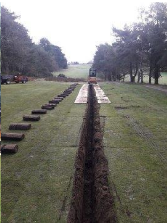
Much needed drainage on the 9 th tee (100m of new drainage)
